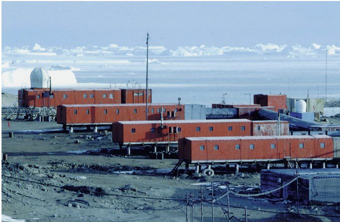
図1 昭和基地居住施設 Fig. 1. Residence building at Syowa Station.
