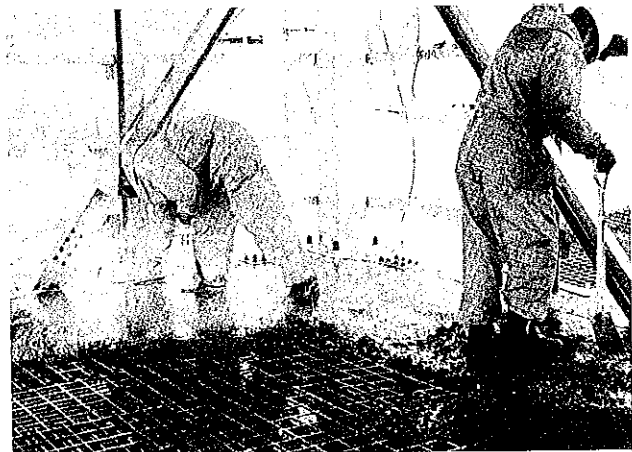
Lattice reinforcement of continuous carbon fibers bonded together with resin was used in the wall footings and floor slabs at Showa Base in Antarctica. The wall footing reinforcement was cut to fit the irregular shape of the rock surface on which the building was constructed.
